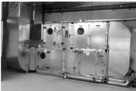
Figure 5: Heat exchanger and humidifier of the supply air
